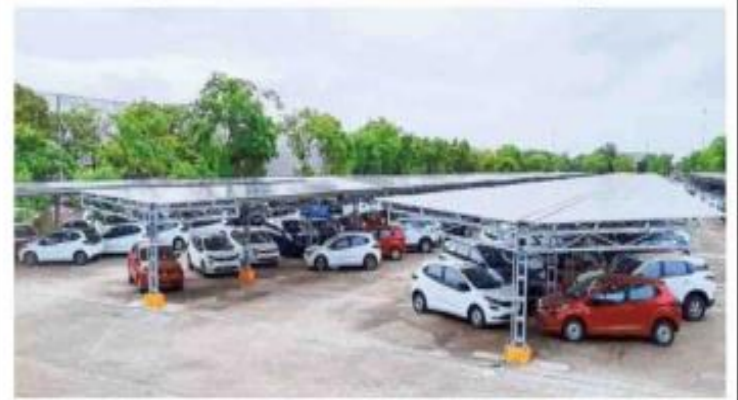
The 6.2 MWp solar carport will generate 86.4 lakh kWh of electricity per year and is estimated to reduce 7,000 tonnes of carbon emissions annually and 1.6 lakh tonnes over its lifecycle
